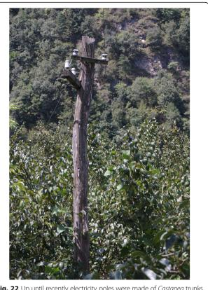
Fig. 22 Up until recently electricity poles were made of Castanea trunks
