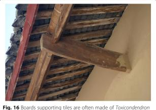
Fig. 16 Boards supporting tiles are often made of *loxicondendron* vernicifluum wood
