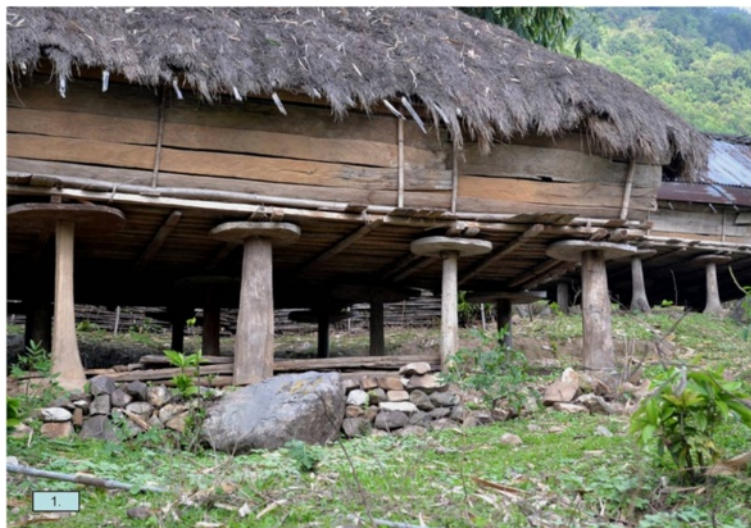
Fig. 1 Large wooden discs that rats cannot pass are placed between the storage house and the pillars it rests on
